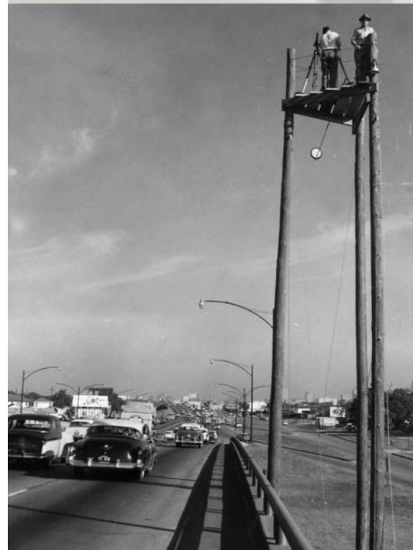
TTI used towers and motion picture cameras to assist in the design, construction, operation and improvement of urban interstates. Shown here is I-45 (the Gulf Freeway) in Houston. (courtesy of TTI Communications)
