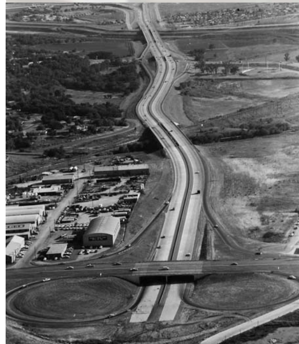
I-35 west weaving through Fort Worth. State Highway 183 crosses the interstate at the bottom of the photo. (courtesy of TxDOT)
