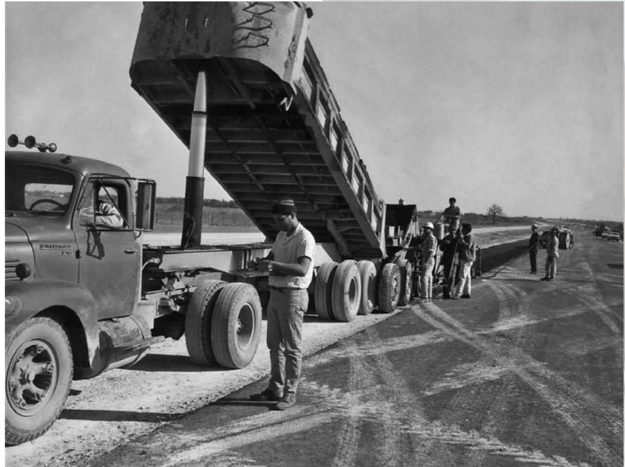
A roadcrew lays an asphaltic base on I-35 south of San Antonio. (courtesy of TxDOT)
