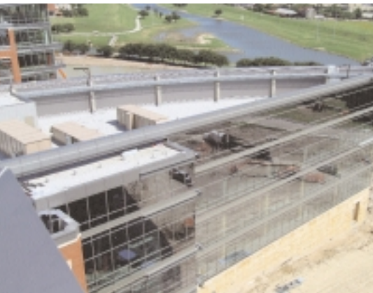
TOP: Views from the Trinity River reveal a different design than the masonry used on the building sides facing the central business district. These curtain walls of glass optimize employee views of the river and landscaped greenway.
